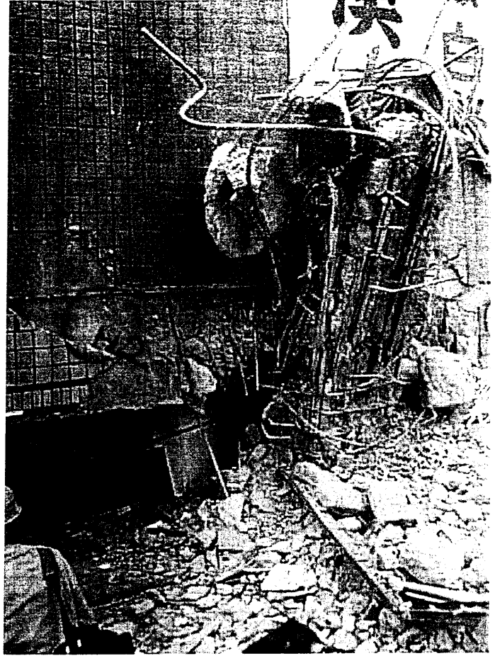
Figure 6 Failure of badly detailed RC columns
